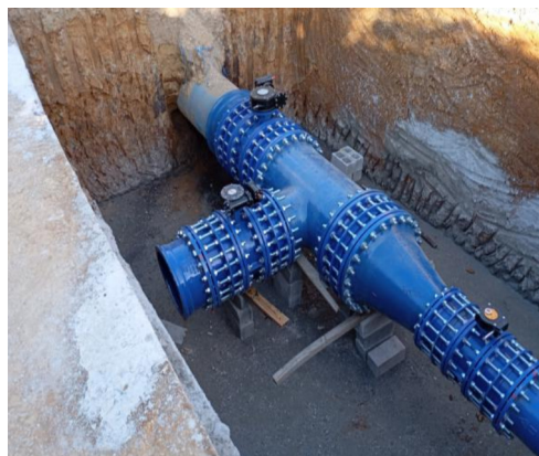
Shut-off valves (PN16atm) for network isolation
